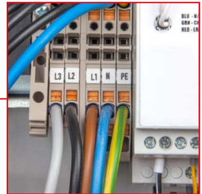
3-phase supply (L3, L2, L1, N, PE)
